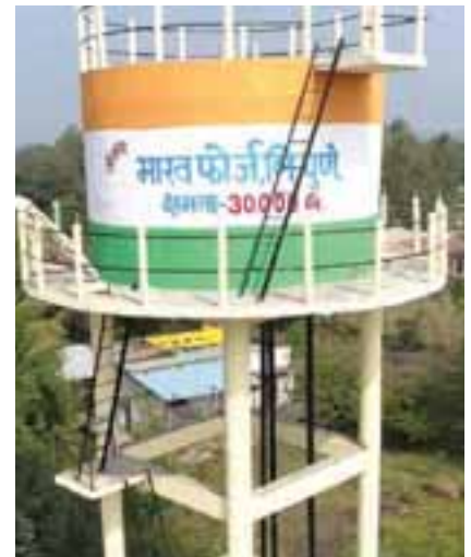
Constructed Drinking Water Tank District: Satara
